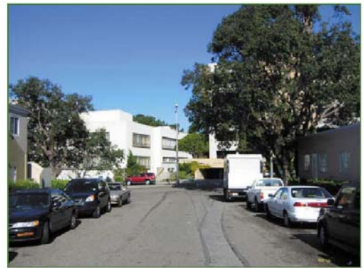
D. View from Cardenas Avenue, looking North towards the Administration building complex
